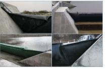
**Variable side slope**Rubber dam can be installed in rivers with any side slope angle up to 90° degree vertical.
