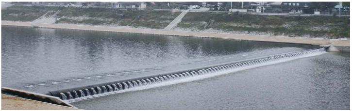
Longer Span Without Piers or Abutment : Rubber dam can be installed without a Mid-structure up to 150m(500ft) in length.
